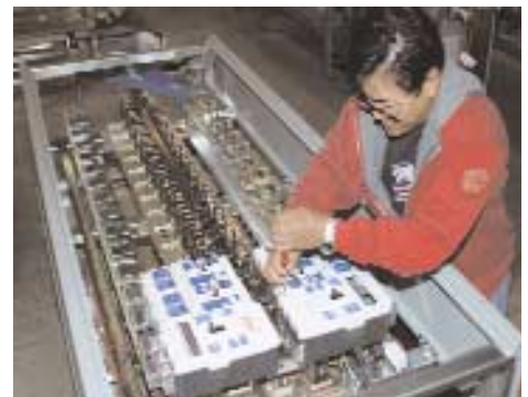
The Assembly of a custom-made Switchboard
